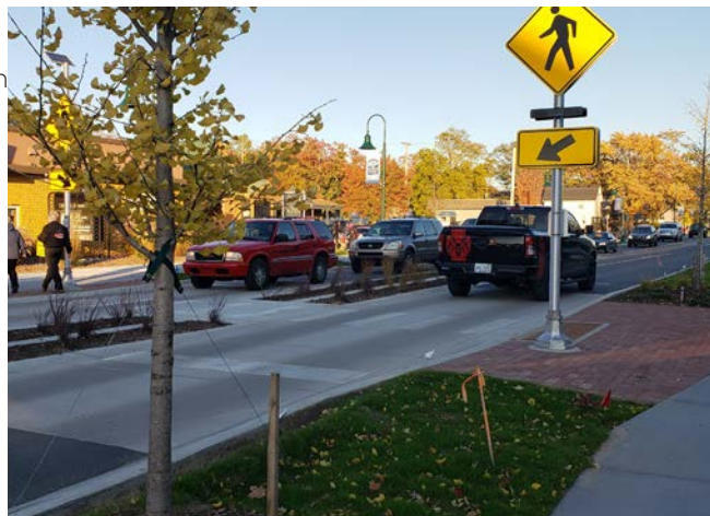
City of Traverse City 8th Street Reconstruction
