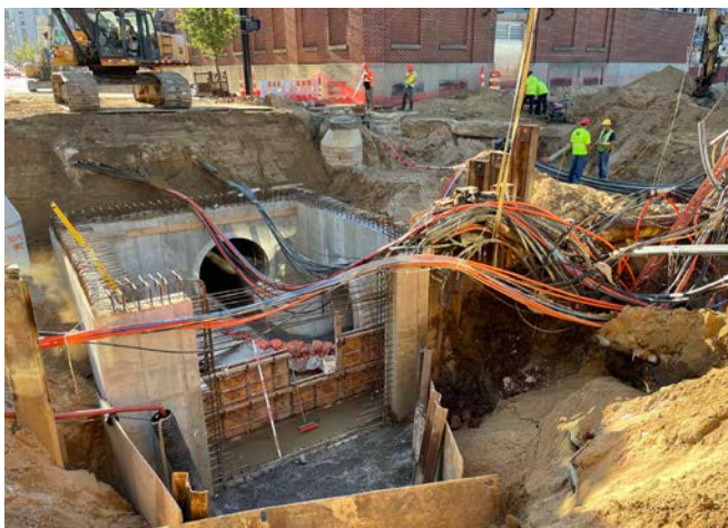
City of Grand Rapids Market Avenue Sewer Relocation
