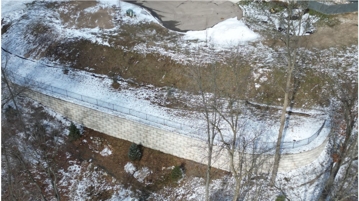
2026 Aerial of Existing Retaining Wall
