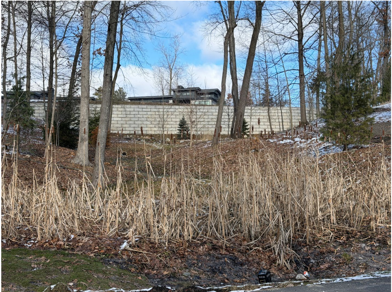
2026 Retaining Wall view from Thornapple River Drive
