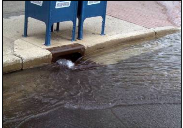
Storm water runoff entering the storm sewer after a rainstorm.
